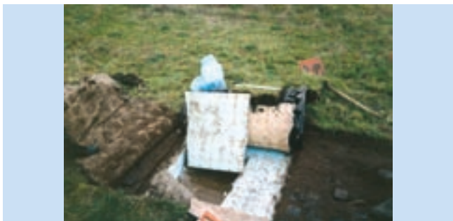
Slika 6: Primer plošč ROOFMATE XPS z zelene strehe (Foto: Dow Building Solutions)
