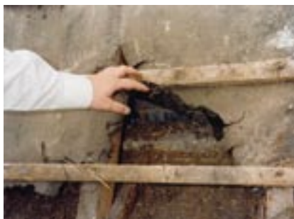
Lomljiva in raztrgana bitumenska membrana
