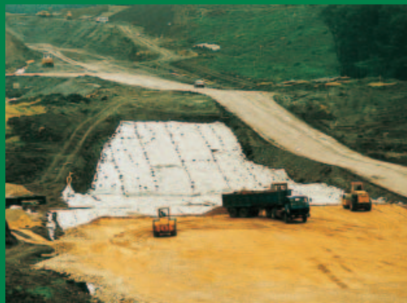
Highway construction (France)
