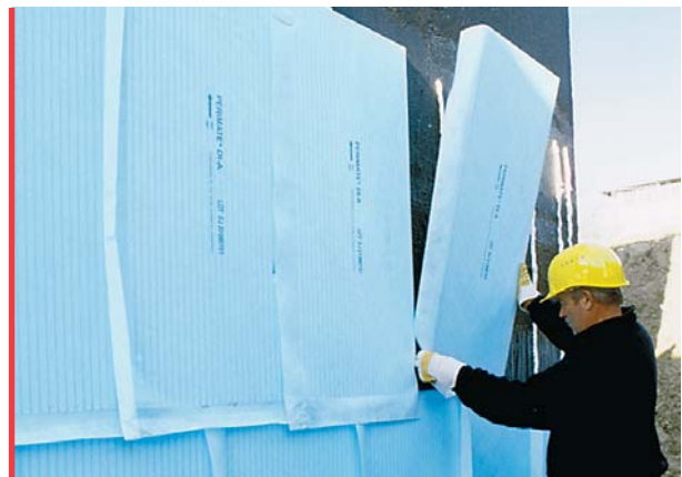
Installing of PERIMATE™ DI-A insulation boards
