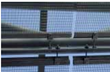
Woven wire cloth elements tensioned using tension profile and clevis screw system
