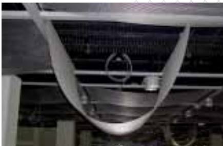
Open position of a woven wire cloth element edged with slotted profiles
