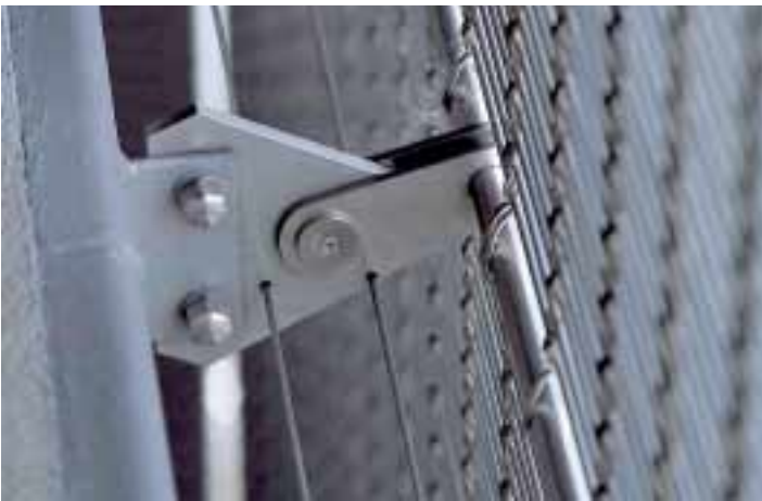
Intermediate fixing: Round bar with integral pendular fixing plates attached to triangular bracket (Type of weave: MULTI-BARRETTE)
