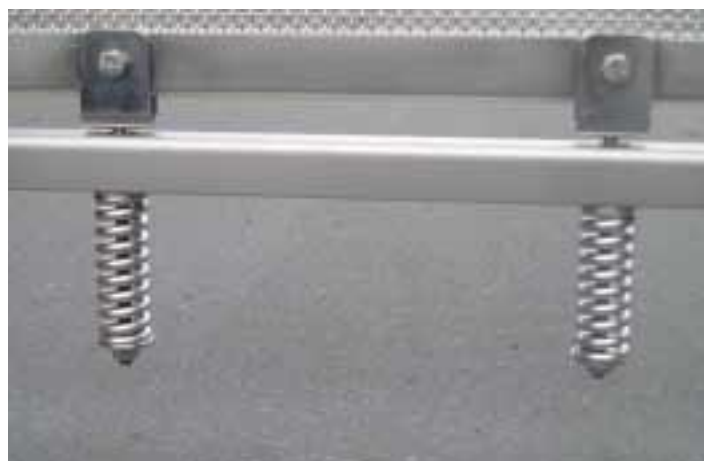
Intermediate fixing: Wire connector
