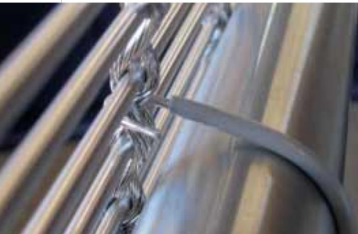
Intermediate fixing: Wire connector
