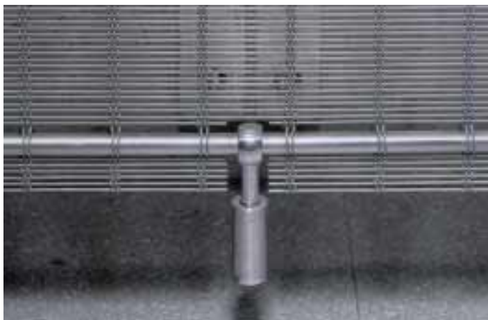
Intermediate fixing: Round bar with integral pendular fixing plates attached to triangular bracket (Type of weave: MULTI-BARRETTE)
